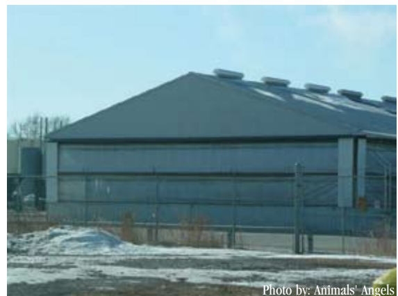
Barn with tarp covered sides to protect against weather.
